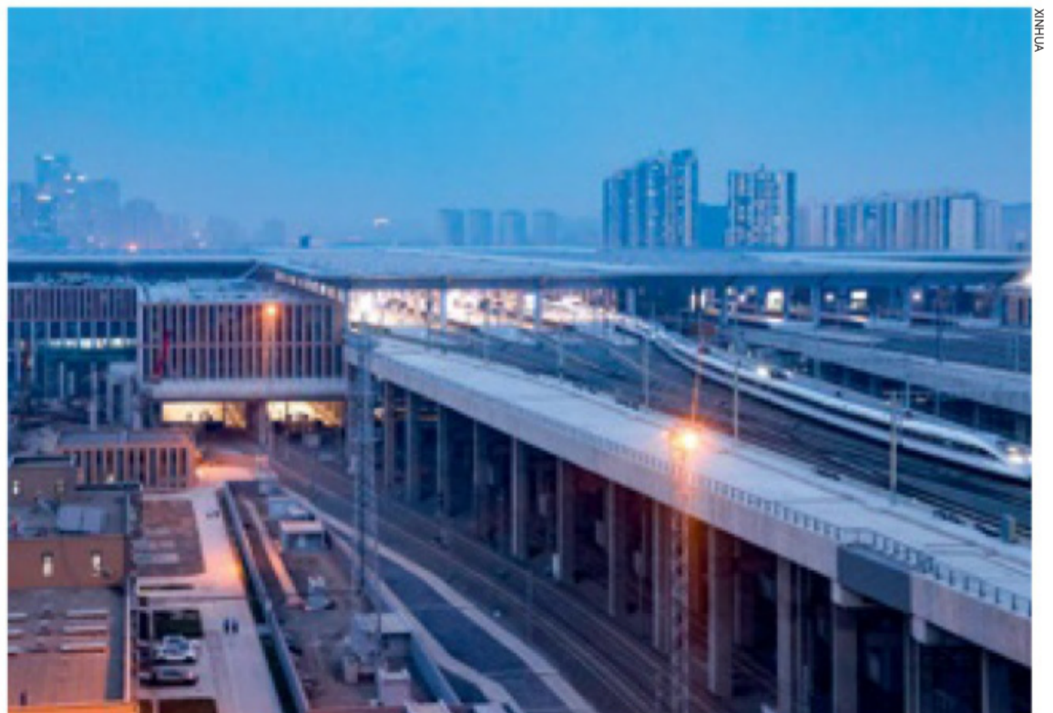
Fengtai Railway Station in Beijing on June 20, the day it reopened after four years of reconstruction. The capital's oldest railway station is now the largest passenger railway hub in Asia
