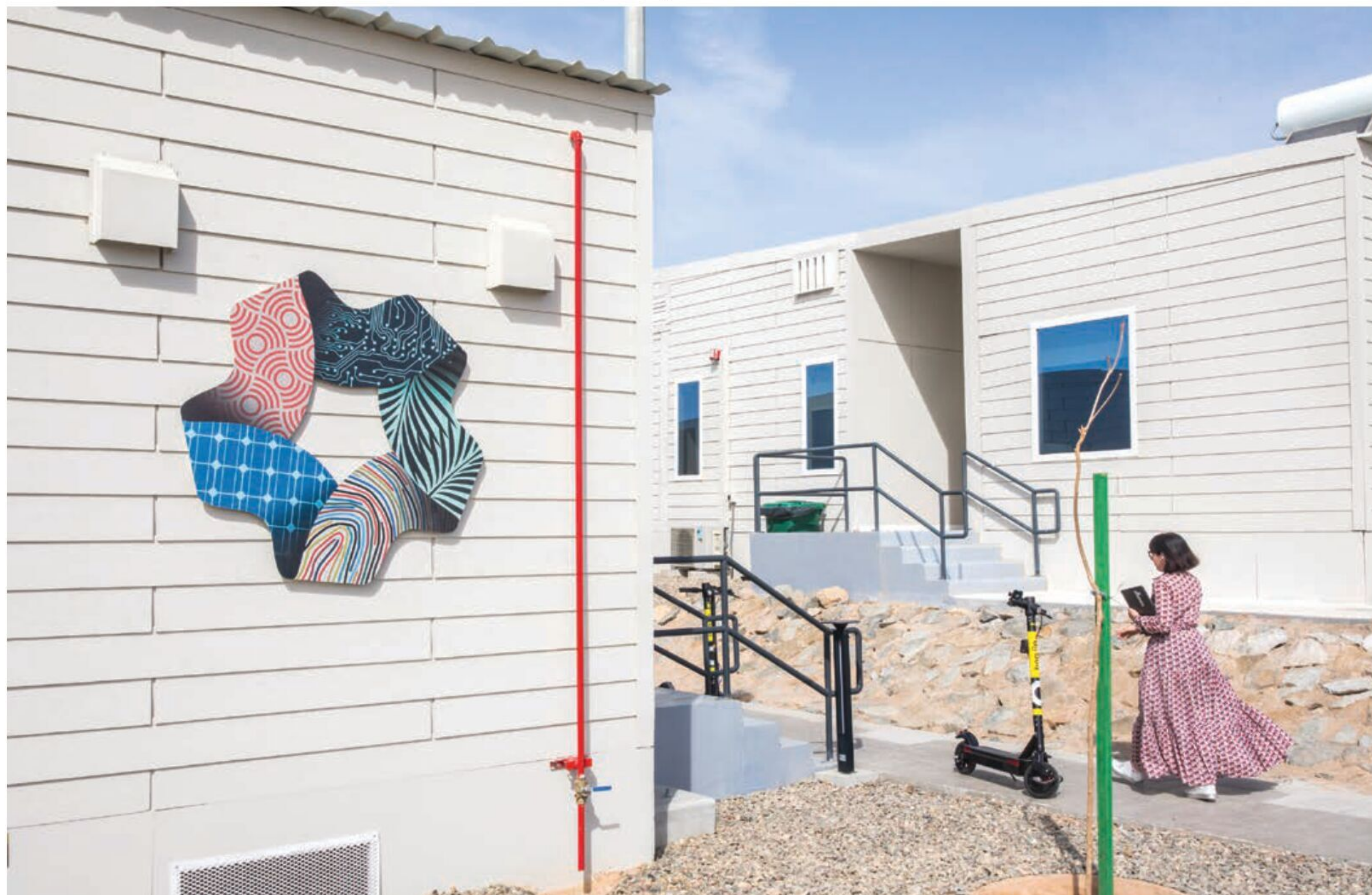
▲ Temporary office buildings
